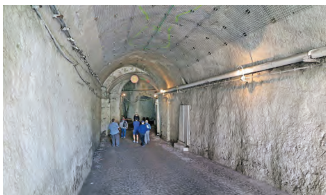
The initial entranceway to Kőbánya has a cobbled floor and recent roof protection
